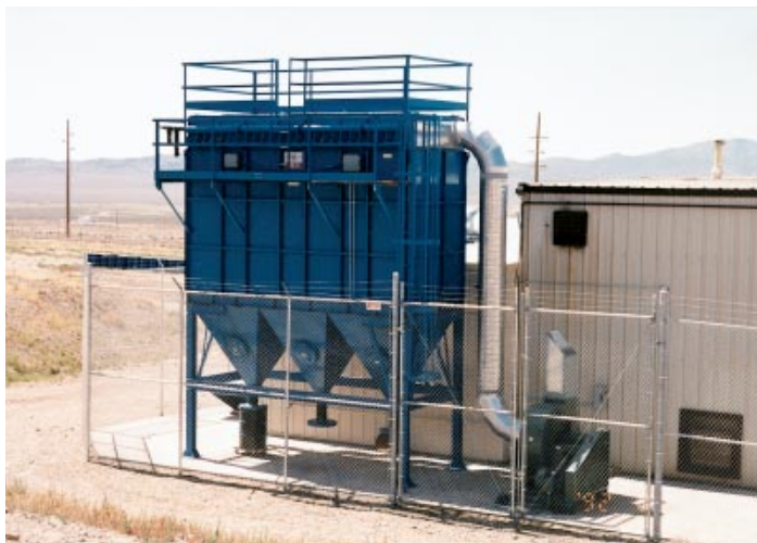
Two TubeJet collectors vent sand handling operations at this foundry. Each collector is rated for 60,000 ACFM.
