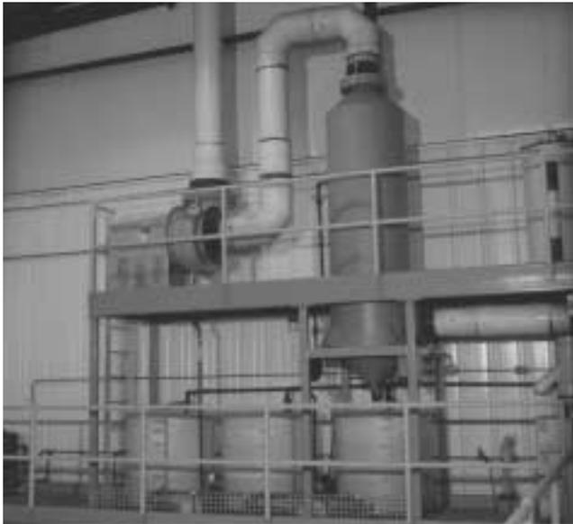
**Gas Scrubber Removes Hazardous Vapors** — An Impinjet® gas scrubber has been employed by a major producer of industrial chemicals to remove hazardous (noxious) vapors. The scrubber vents both bottle filling and dry bulk filling areas at the company, which produces hydrochloric, sulfuric and nitric acid as well as formaldehyde and ammonia.
